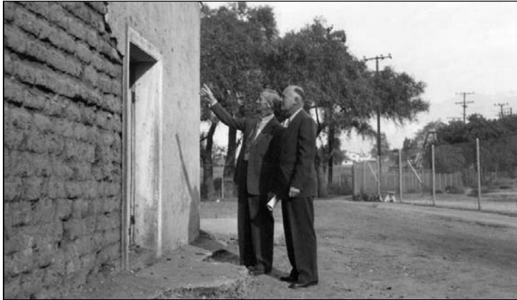
Figure 13: Detail of east elevation (San Marino Historical Society, 1952)
