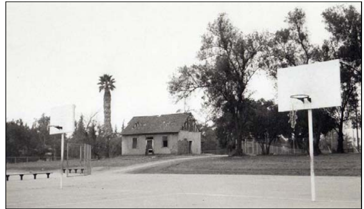
Figure 16: South and east elevations, view northwest (San Marino Historical Society, 1952)
