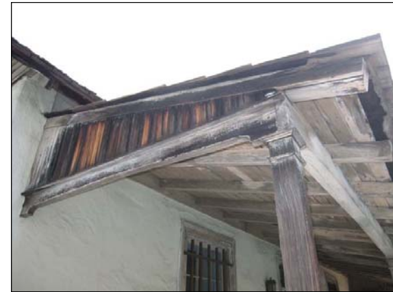
Figure 37: Detail of porch roof along south elevation, view west (CA, 2009)
