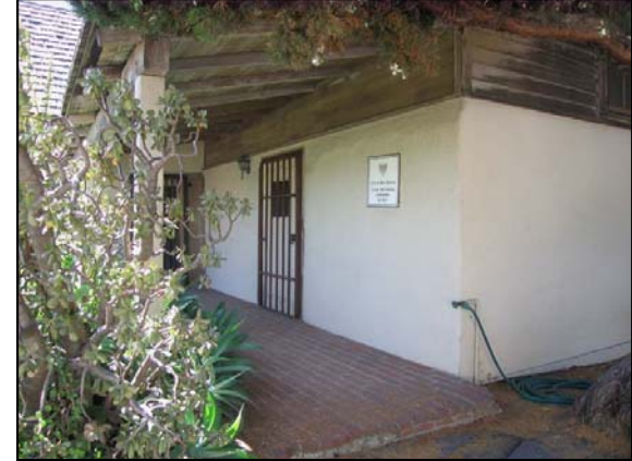
Figure 32: Detail of porch along east elevation, south wing, view south-east (SMSD, 2008)
