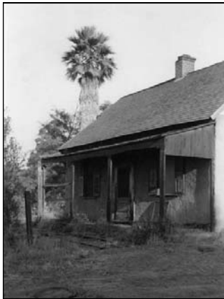
Figure 10: South elevation, view northwest (San Marino Historical Society, 1947)
