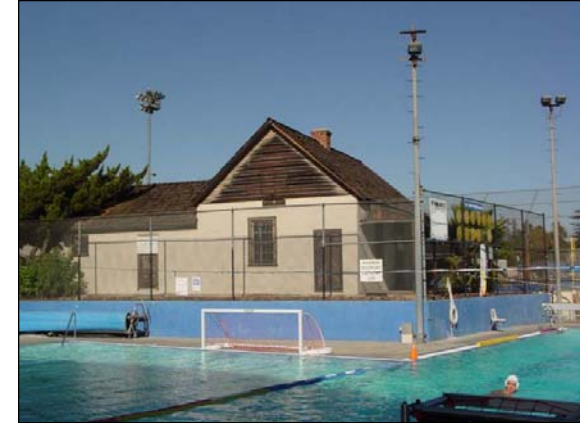
Figure 33: West elevation, north wing (left) and south wing (right), view northeast across pool (CA, 2008)
