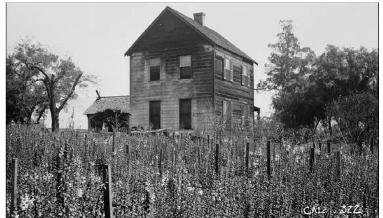
Figure 4: West elevation, view northeast (Historic American Building Survey, 1936)
