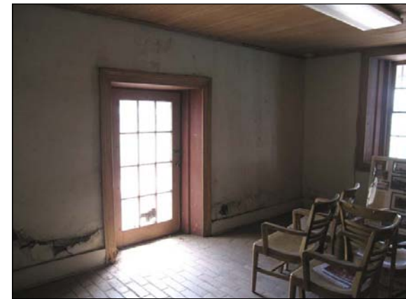
Figure 53: Interior of south wing, east room, view southeast (CA, 2009)
