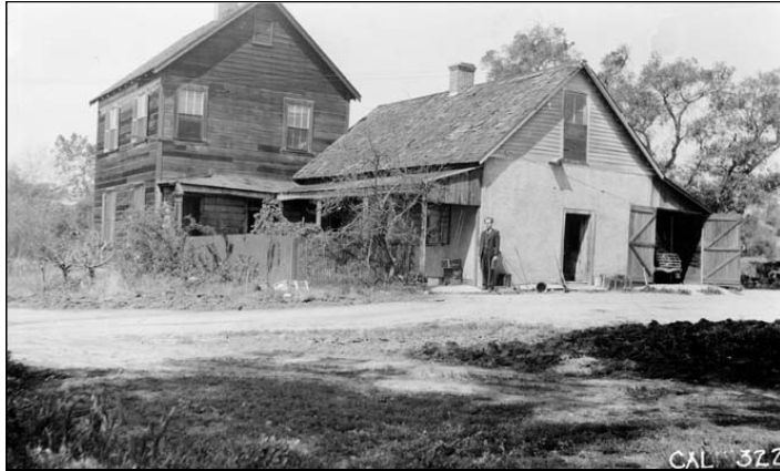
Figure 1: South elevation (left) and north elevation of south wing (right), note two story wood frame addition, view northwest (Historic American Building Survey, 1936)
