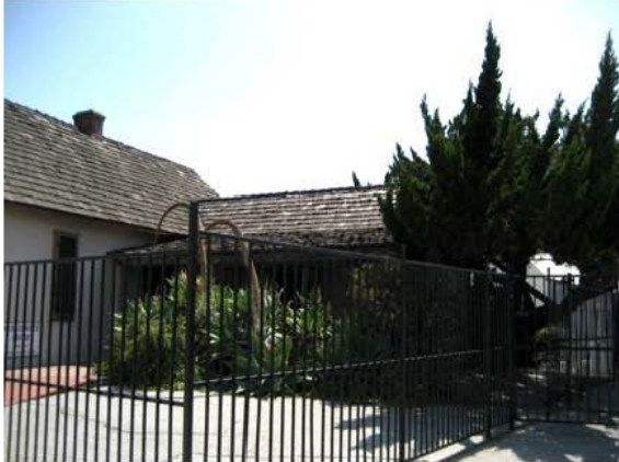
Photo 2 - Northeast view of the structure.
