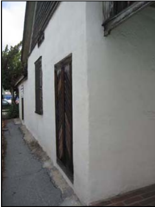
Figure 39: West elevation, south wing (foreground) and north wing (background), view northeast (CA, 2009)
