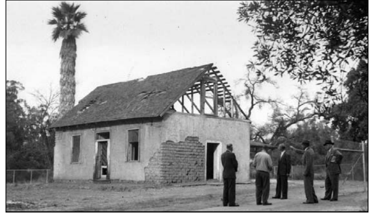
Figure 12: South and east elevations, view northwest (San Marino Historical Society, 1952)
