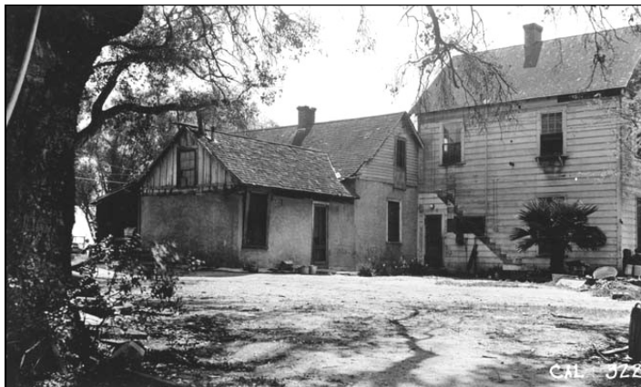
Figure 2: North elevation (left) and south elevation (right), note two story wood frame addition, view southeast (Los Angeles Public Library, 1936)
