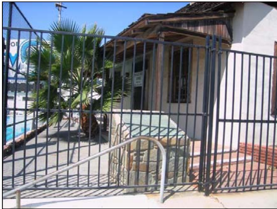
Figure 35: Detail of porch along south elevation, south wing, view west (SMSD, 2008)
