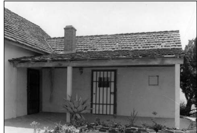
Figure 19: East elevation corredores, view west (San Marino Historical Society, nd)
