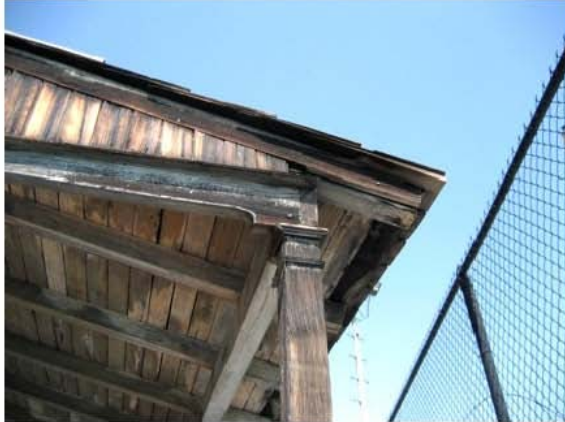
Photo 6 - Detail of trim at south porch.
