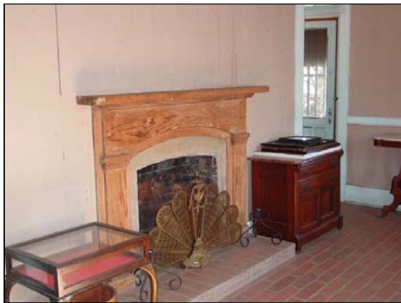
Figure 51: Fireplace in south wing, west room, view southeast, note door to south elevation porch (CA, 2008)
