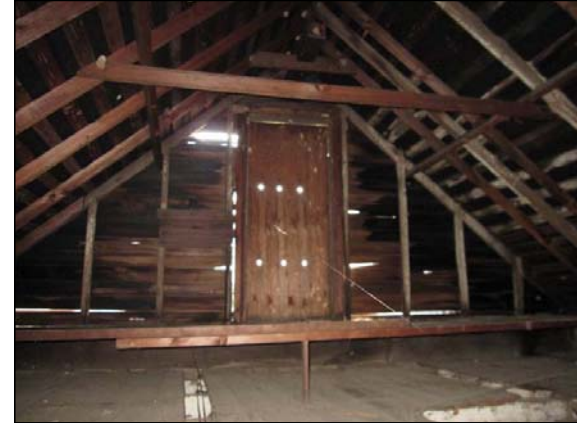
Figure 57: South wing attic, view east, note contemporary roof framing (CA, 2009)
