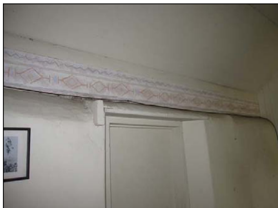
Figure 46: Detail of north wing, view west (CA, 2009)
