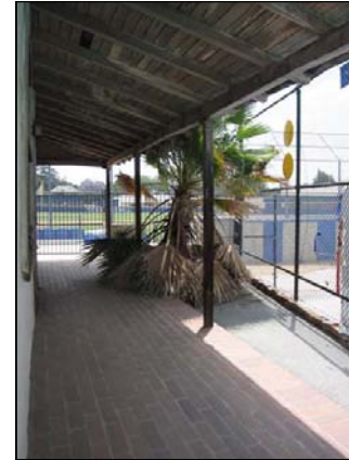
Figure 36: Porch along south elevation, south wing, view east (CA, 2009)
