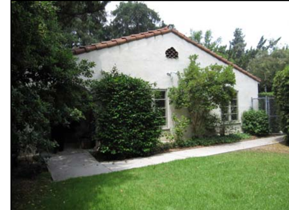
Figure 75: East elevation of Thurnher House, view west (CA, 2009)
