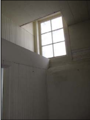
Figure 43: Detail of window on north wing, view northwest (CA, 2009)
