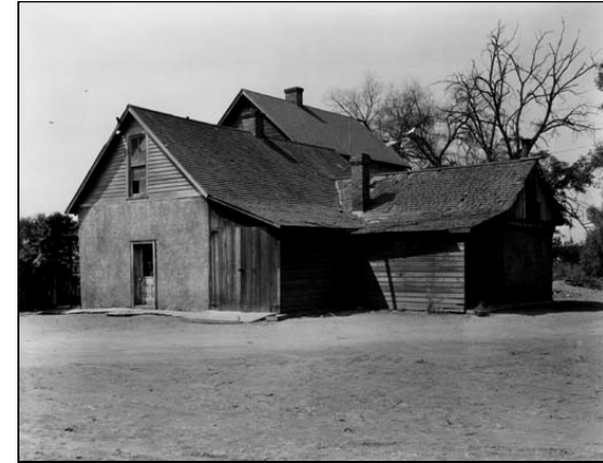
Figure 7: East elevation, view southwest (Los Angeles Public Library, nd)
