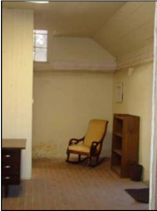
Figure 42: Interior of north wing, view northeast (CA, 2008)
