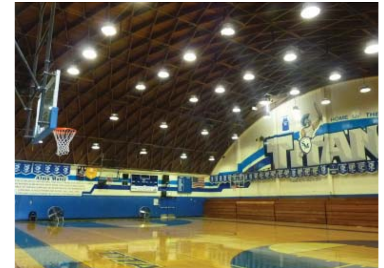
San Marino High School Large Gymnasium
