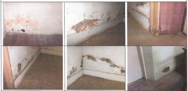
The photos above indicate significant water damage to the interior portions of the building, including ceiling areas. It is not apparent the effect water damage has had to the structural integrity of the building.
