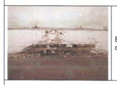
Base board areas have indications of significant termite damage.
